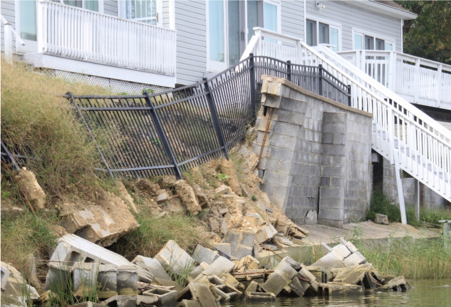
Eventual Collapse of Retaining Wall (July 2018)
