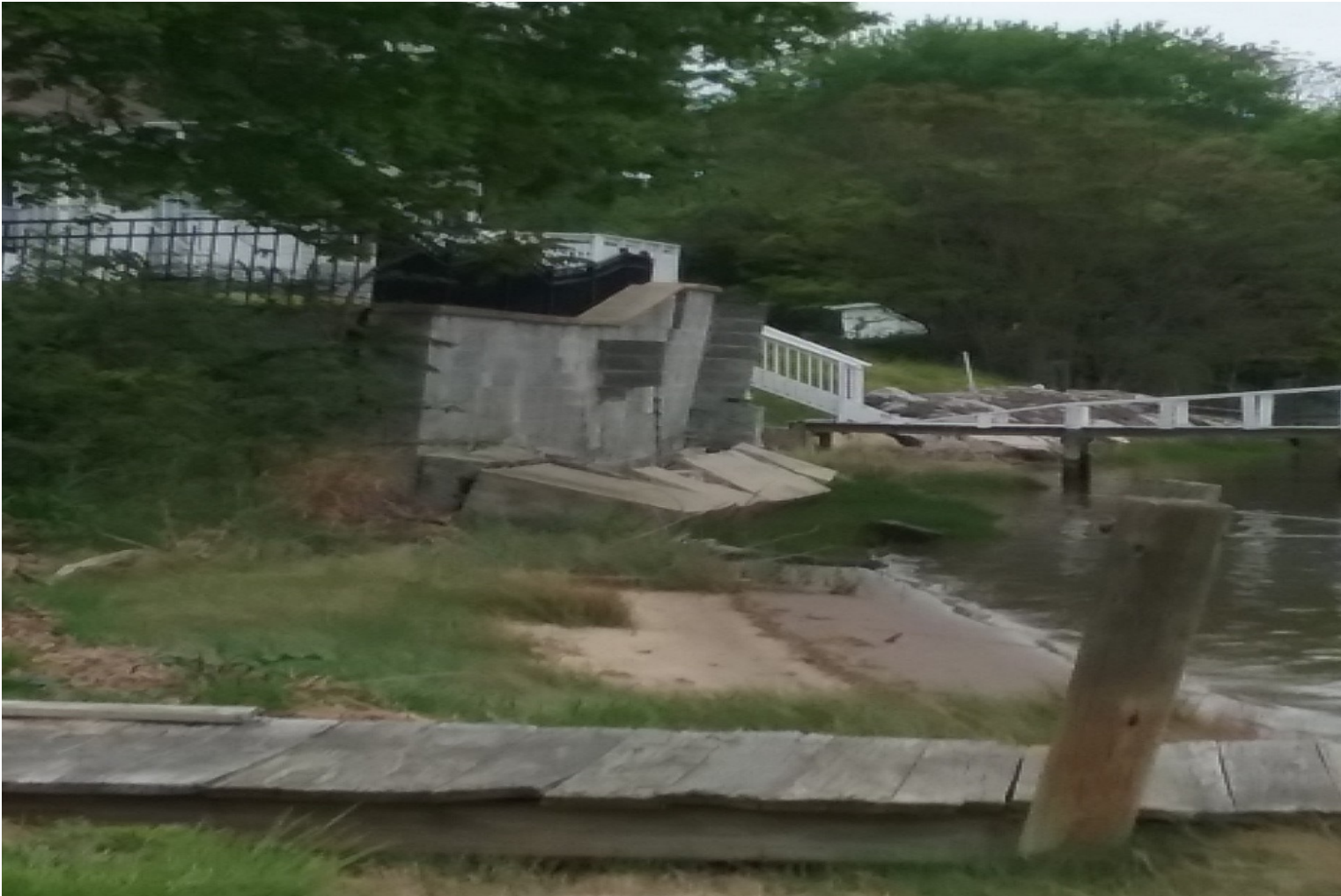
Retaining Wall Showing at Risk of Collapse (May 2018)
